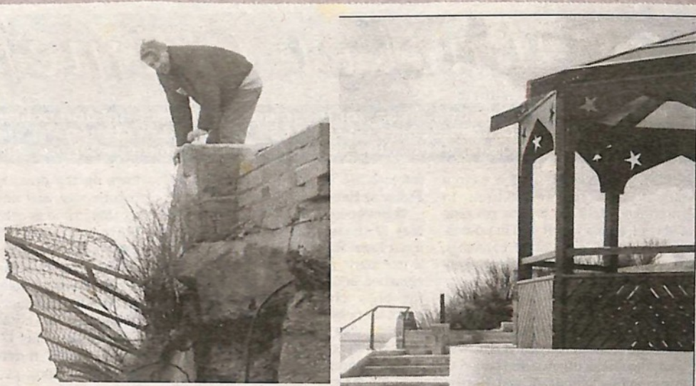
□ ABOVE: Richard Palmer inspects the damage caused by the storm in 1997
